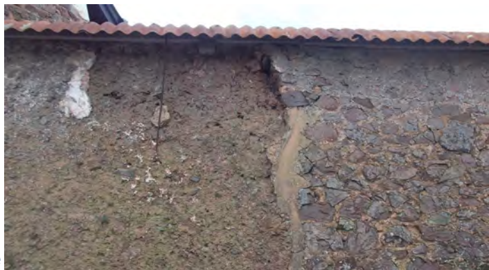
Figure 32 (above): Stone and Cob boundary walls
